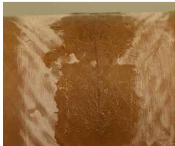
*Curing or hardening in a matter of minutes, the “patches” or “tabs” secure the pipe sections in the proper alignment*
