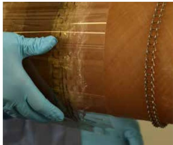
*Gently press the weld strip around the surface of the pipe joint until the ends overlap; lightly press out the air bubbles with gloved hands*
