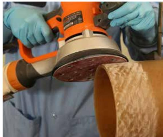
*Roughen the outside surfaces with a sander approximately 3 cm (1 in) farther in from the ends than the finished weld surface; where inside welds are possible, interior surfaces should be sanded prior to assembly*
